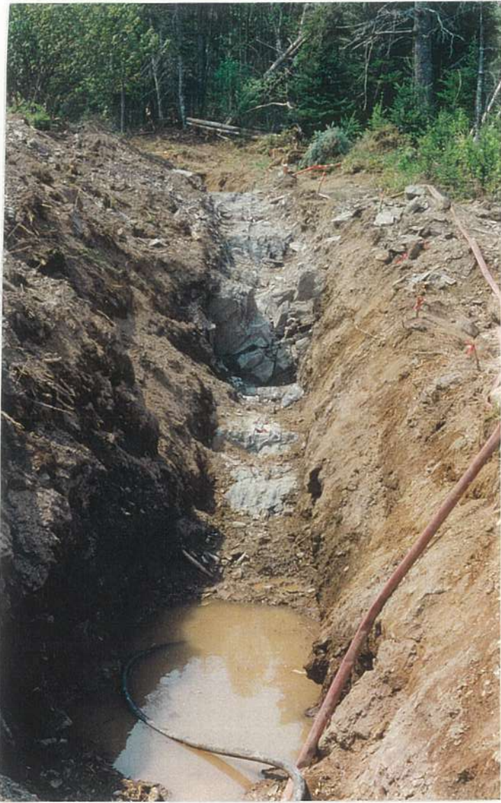
Trench 2, looking northwest, note ridge of the more resistant ribbon sediments
